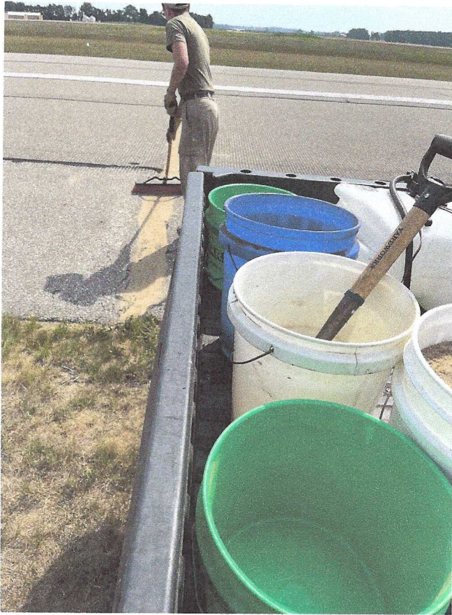
July 31, 2026 – filling cracks with fine sand on Runway 18/36
