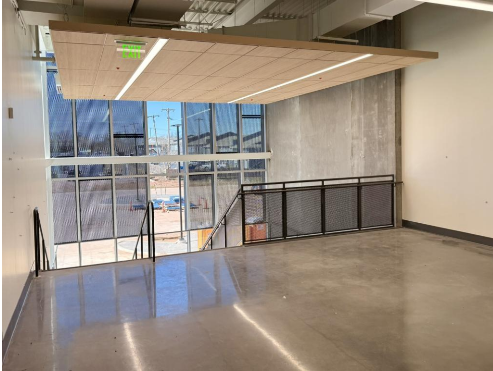
WEST STAIRWELL WOOD CEILING
