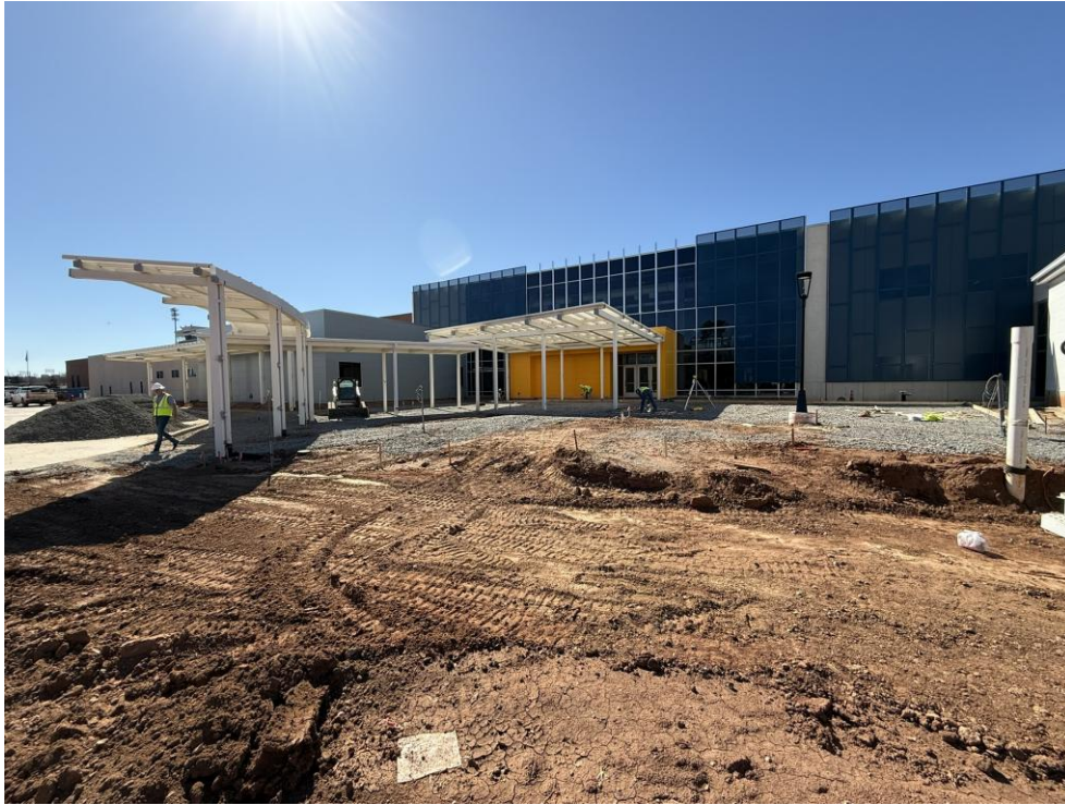
EXTERIOR – BUS DROP-OFF / PIONEER PLAZA / SECONDARY ENTRY
