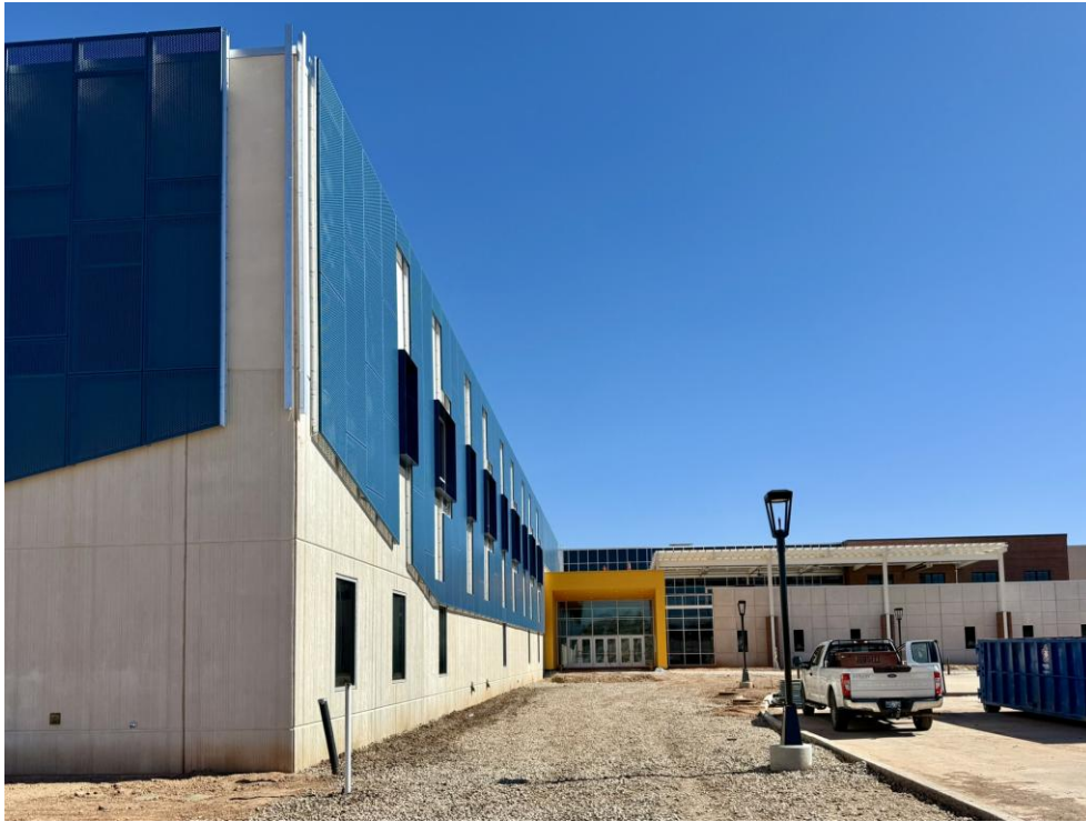
EXTERIOR – MAIN ENTRY
