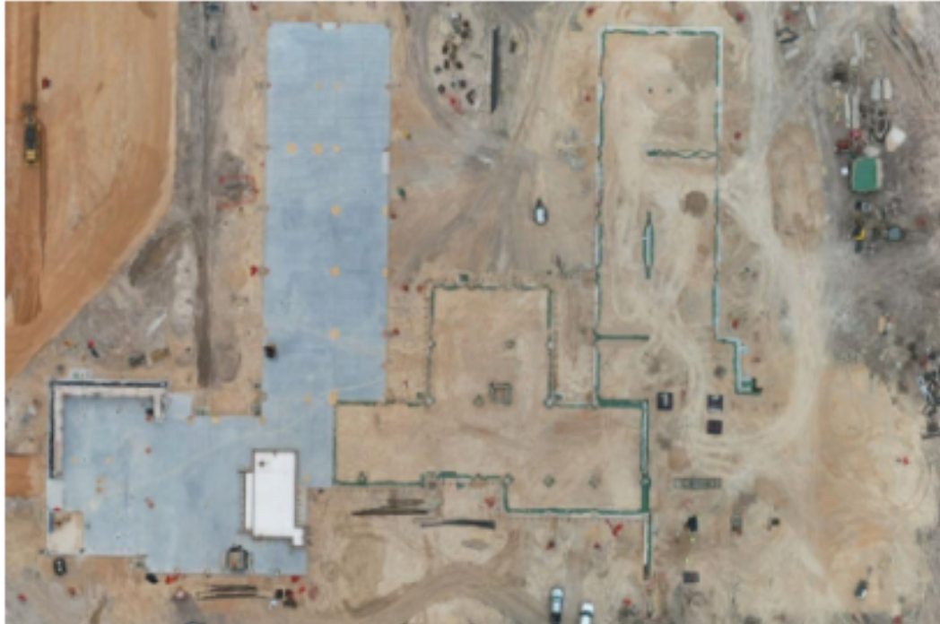
Aerial View of Building Pad
