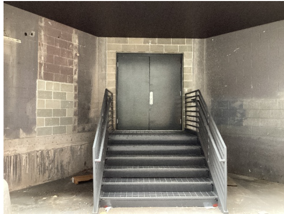
New Exterior Stairs in the Alley
