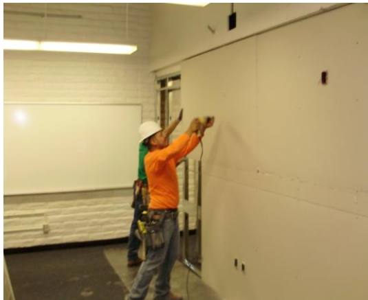
Elementary Pod Air-wall Replacement
