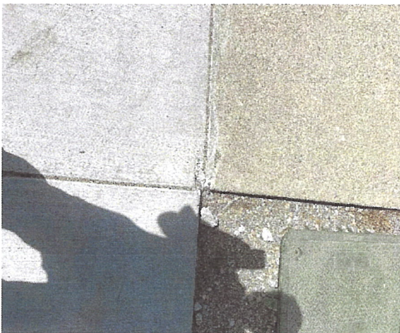
Fig. 1 - Concrete spatter
