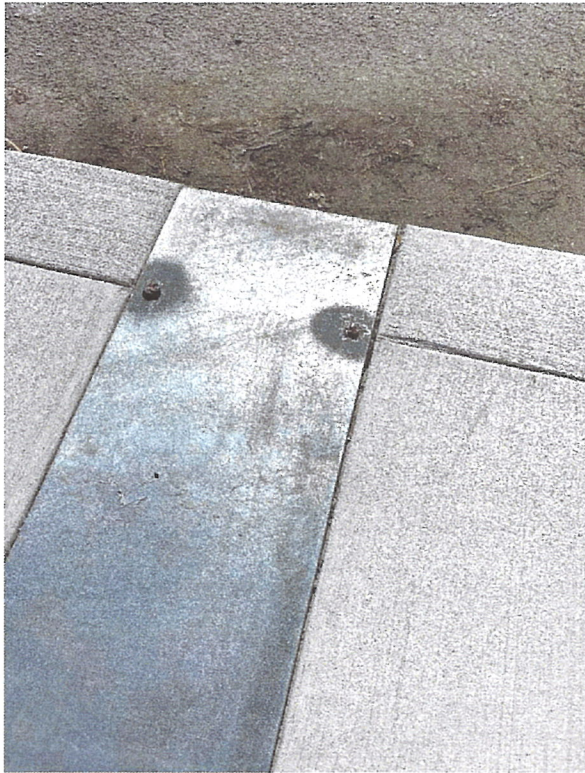
Fig. 7 – Protruding fasteners
