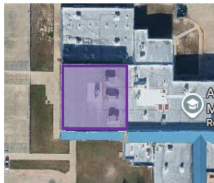
Figures 5, Aerial views of Audie Murphy Middle School: Gym roof replacement area
