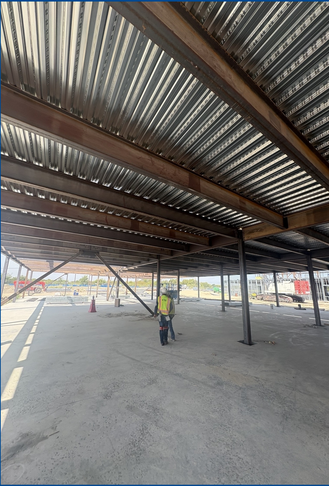
Area F Classroom Wing
