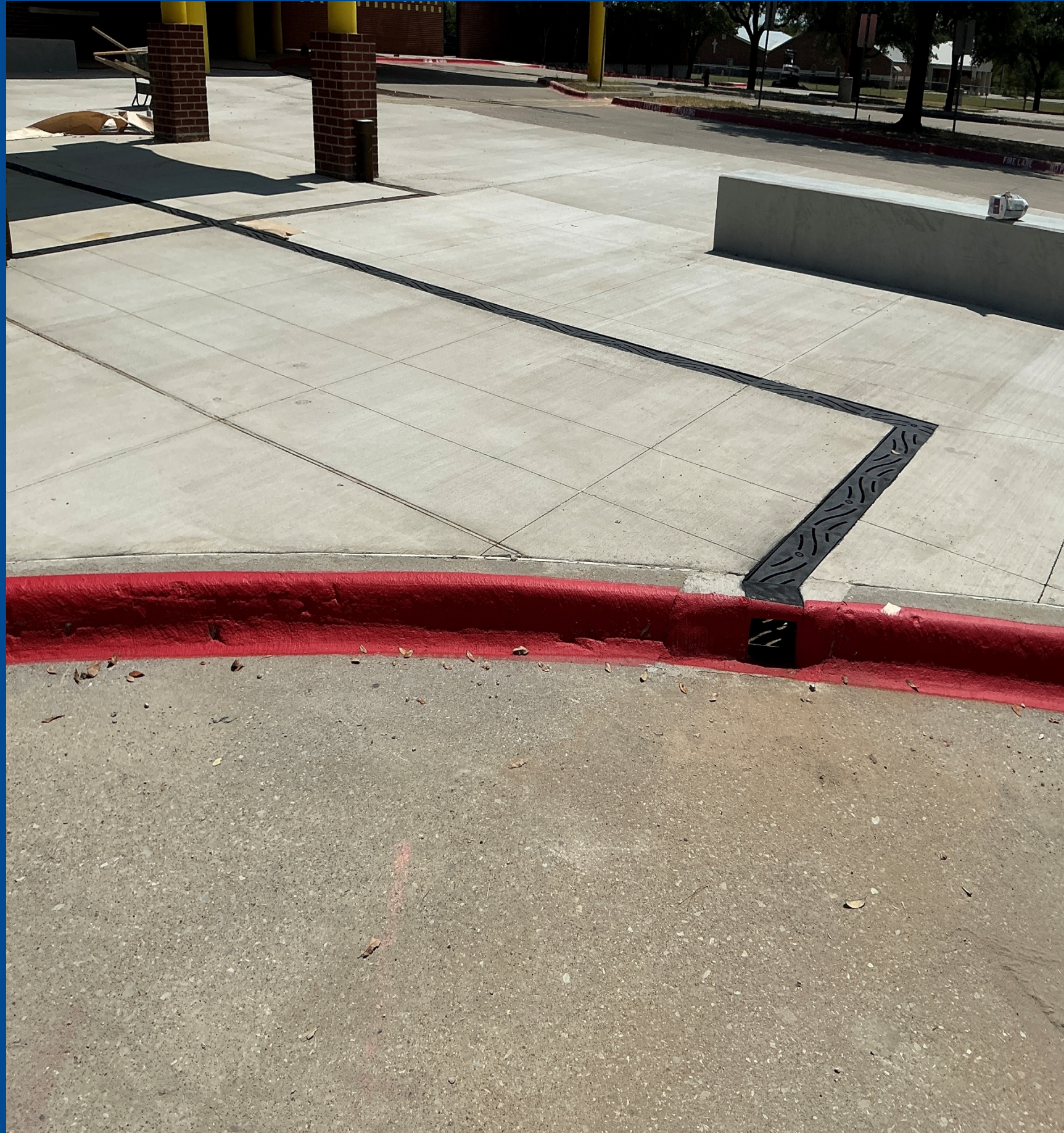
New Entry Sidewalks & Drains
