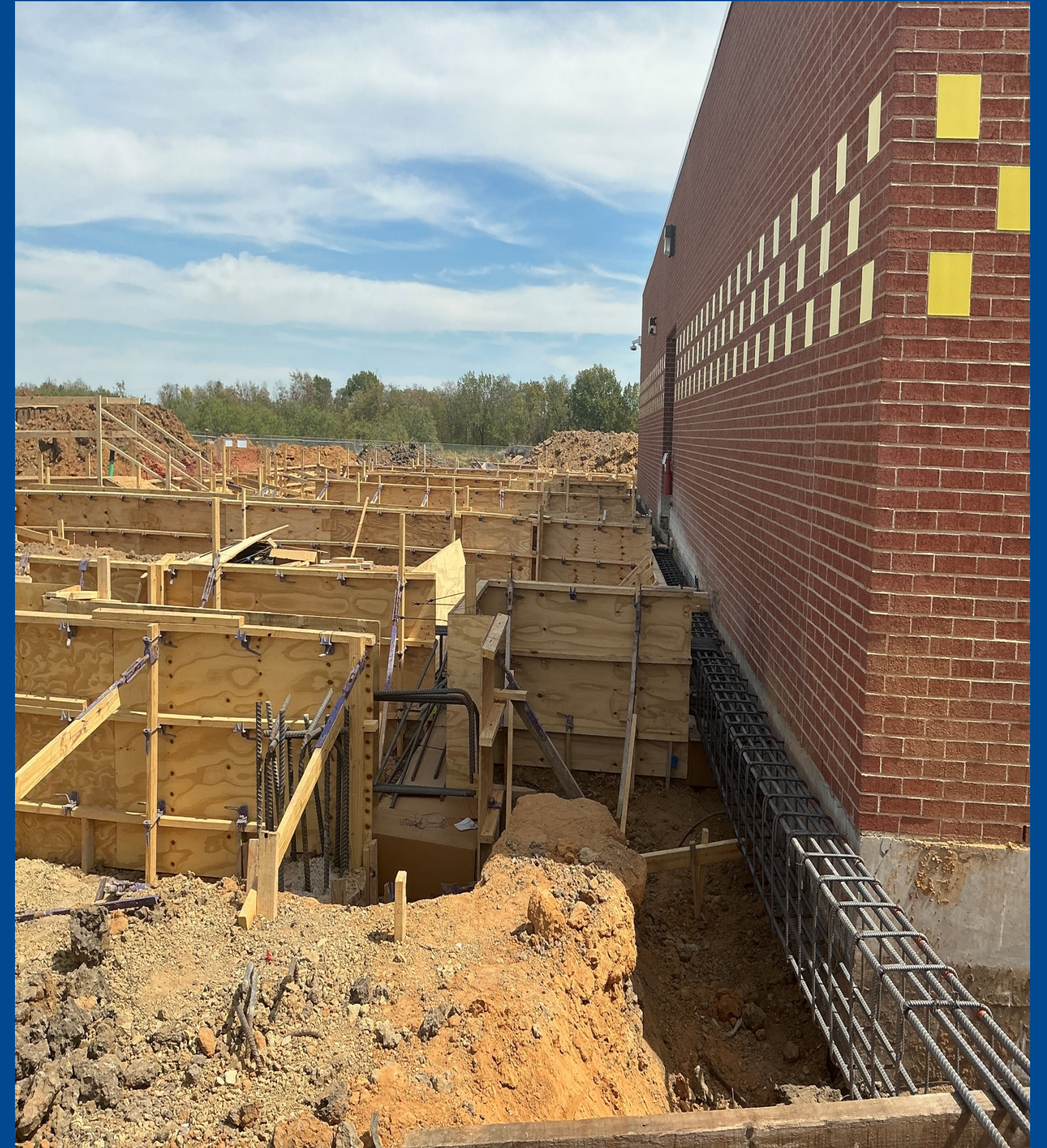
Formed Grade Beams
