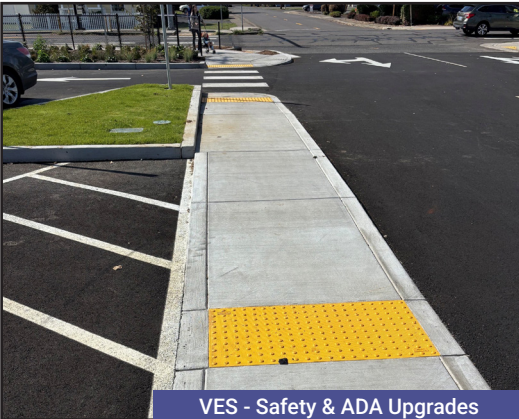
VES - Safety & ADA Upgrades
