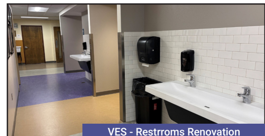
VES - Restrooms Renovation
