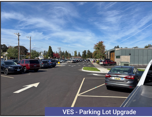
VES - Parking Lot Upgrade
