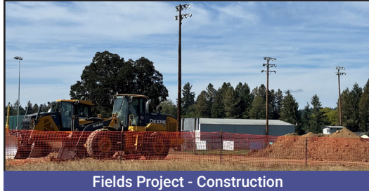
Fields Project - Construction
