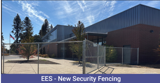
EES - New Security Fencing
