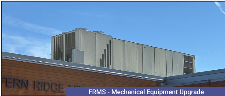
FRMS - Mechanical Equipment Upgrade
