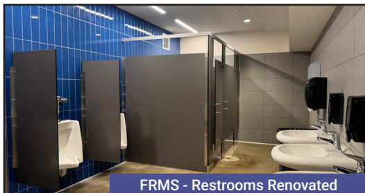
FRMS - Restrooms Renovated
