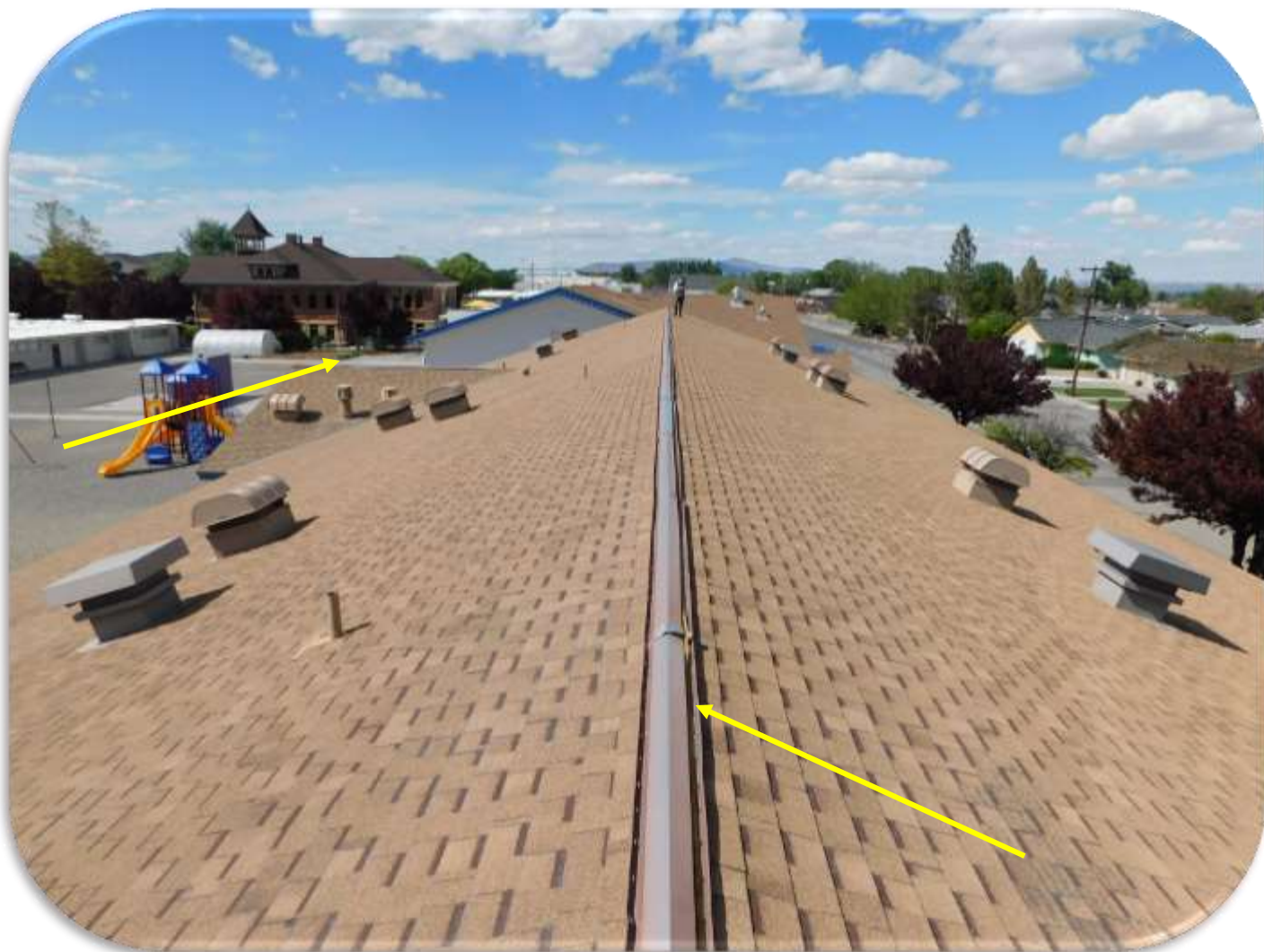
(Y.E.S.), #500 OVERVIEW OF THE MAIN ROOF LOOKING TO THE NORTH. VENTED RIDGES
