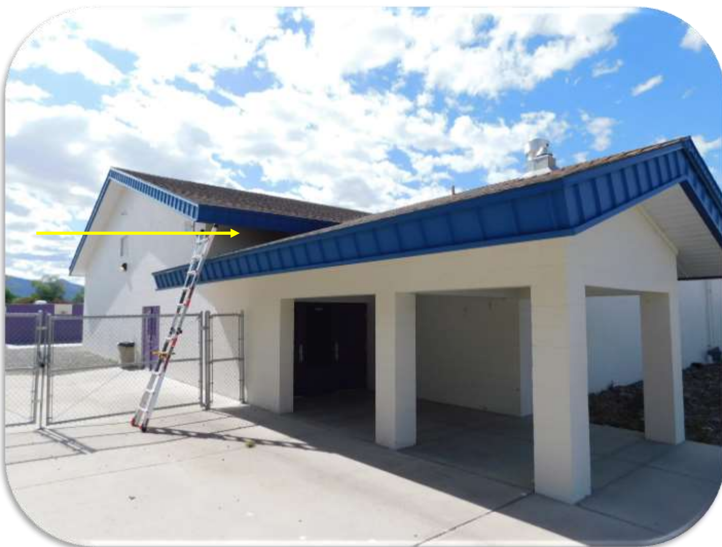
OVERVIEW OF THE MULTI-PURPOSE ROOM BUILDING YERINGTON MAIN ENTRANCE
