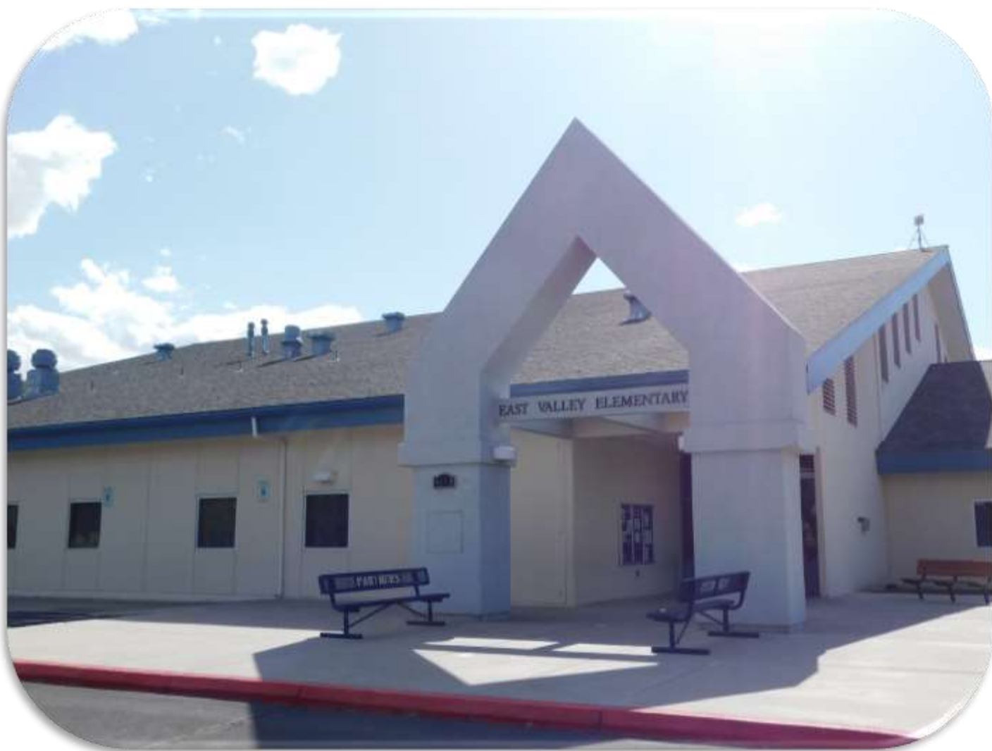
EAST VALLEY ELEMENTARY SCHOOL FRONT ENTRANCE.
