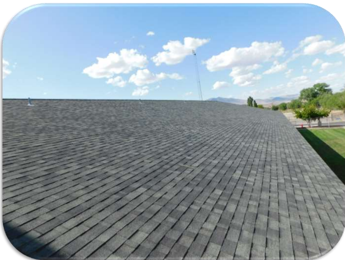
EAST SDIE OF THE BUILDING EAST WING EAST SIDE.
