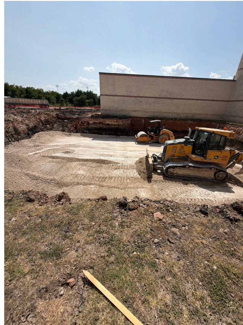
Building Pad Construction
