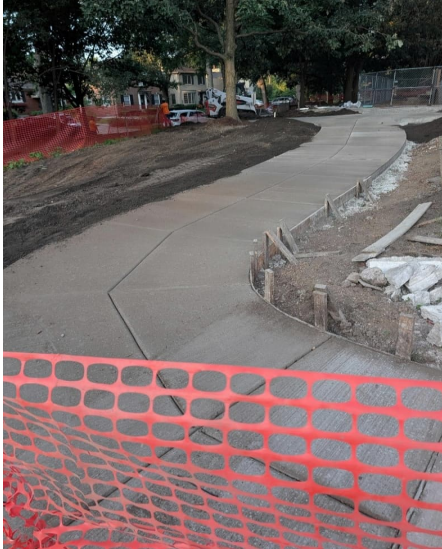
Sidewalks Concrete Poured & Backfilled
