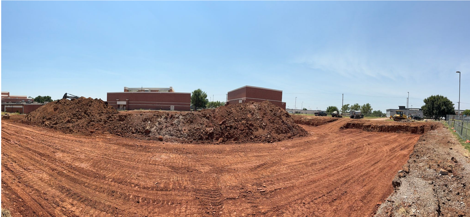
EARTHWORK AT MULTI-SPORT FACILITY
