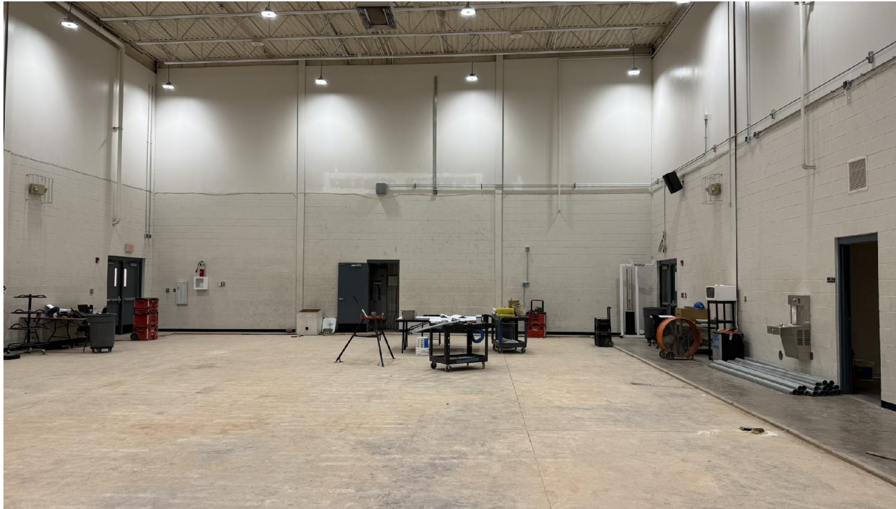
DEMOLITION AT POM_CHEER BUILDING
