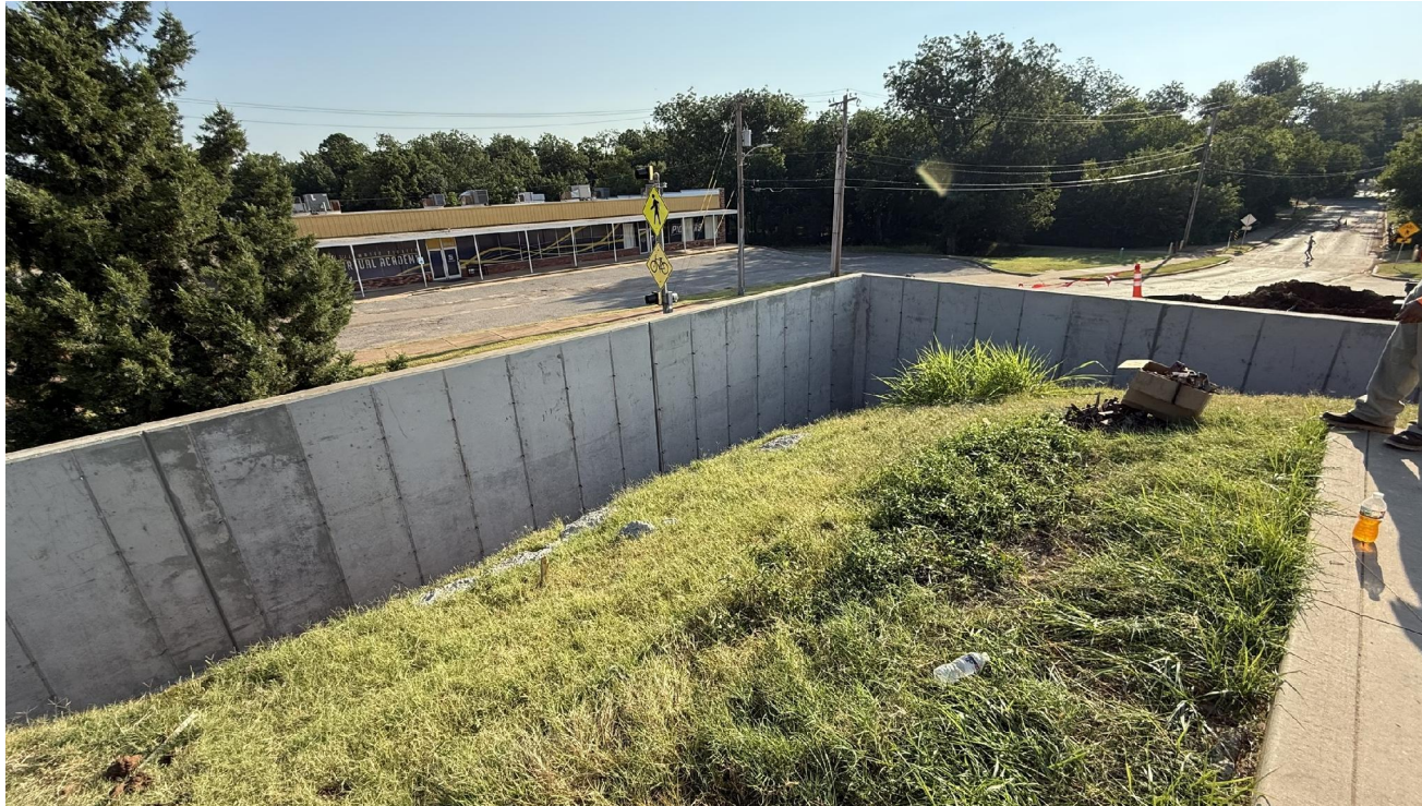
NORTH RETAINING WALL AT POLE VAULT
