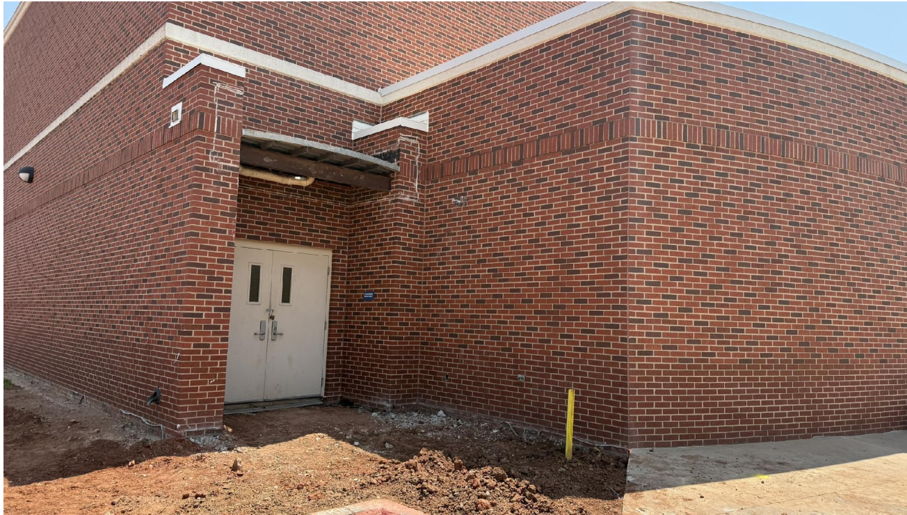
DEMOLITION AT POM_CHEER BUILDING
