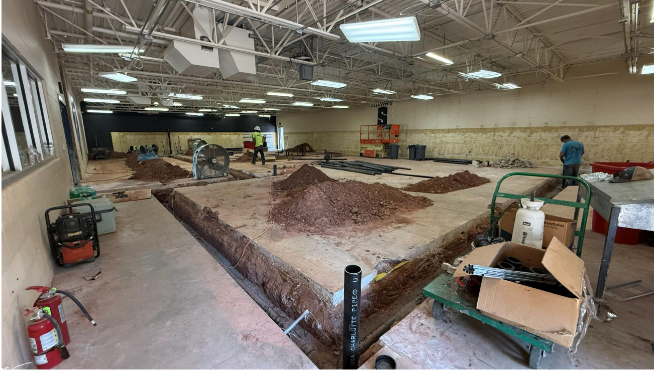
SOCCER_TRACK RENOVATION INTERIOR PLUMBING
