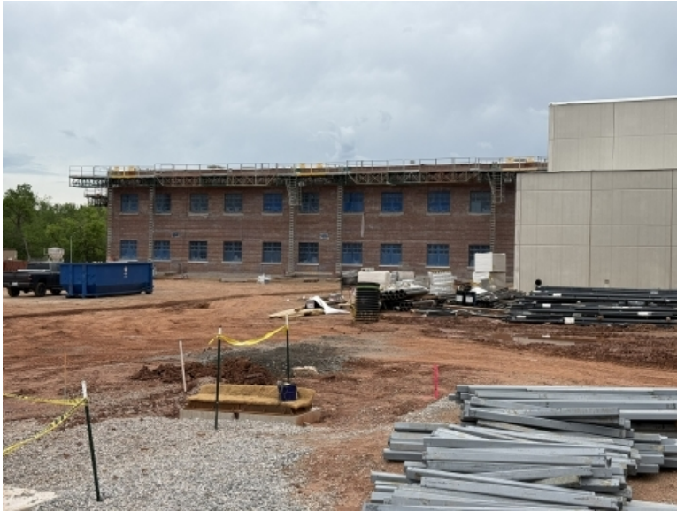
AREA 1 – NW EXTERIOR BRICK SCAFFOLDING
