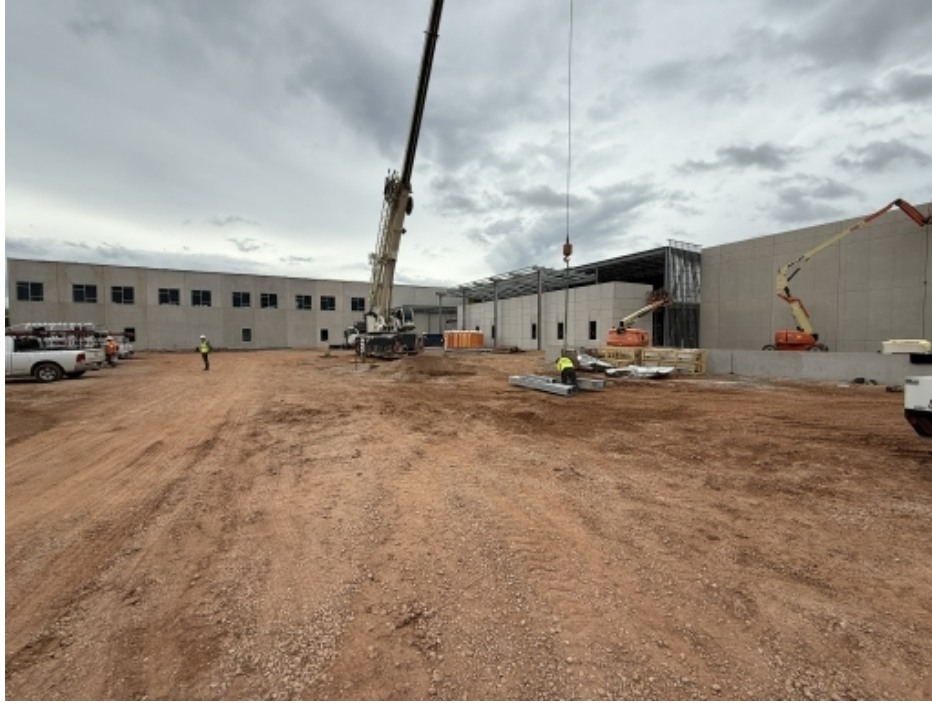
AREA 5 – PRECAST ERECTION
