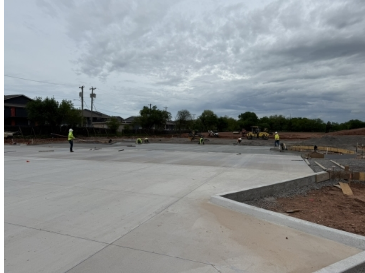
ROUGH GRADING AT NORTH CIMARRON PLAZA AREA
