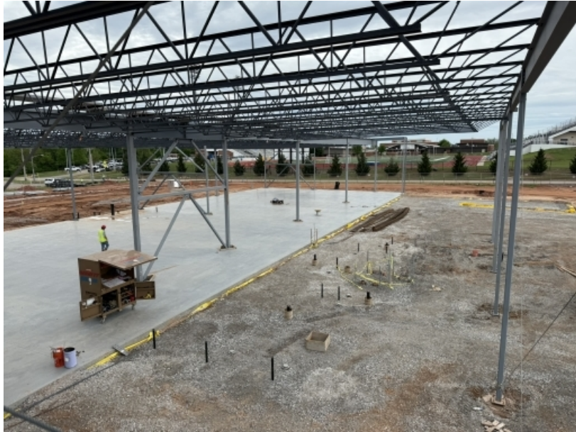
AREA 6 – PW WING STEEL ERECTION AND SLAB
