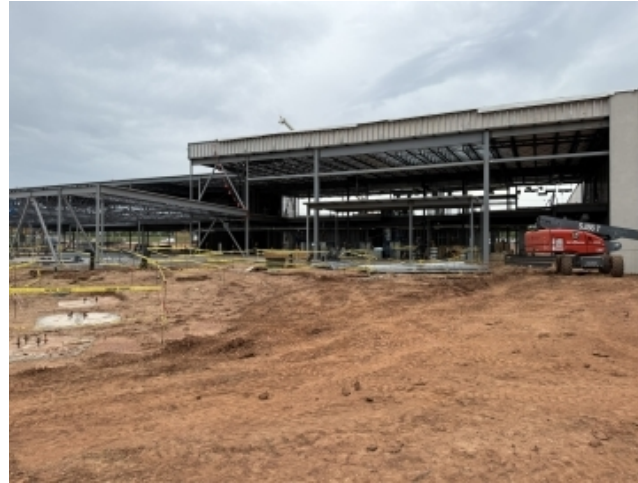
AREA 5 – STEEL ERECTION AT FACS
