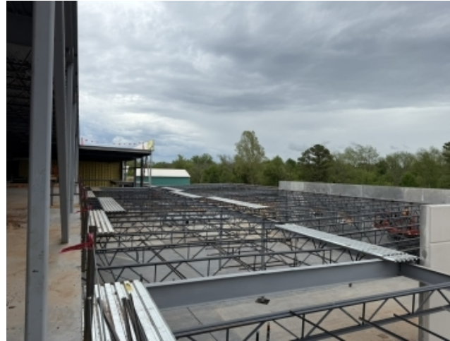
AREA 5 – STEEL ERECTION AT FACS
