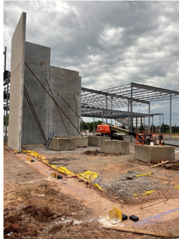
AREA 6 – PRECAST ERECTION
