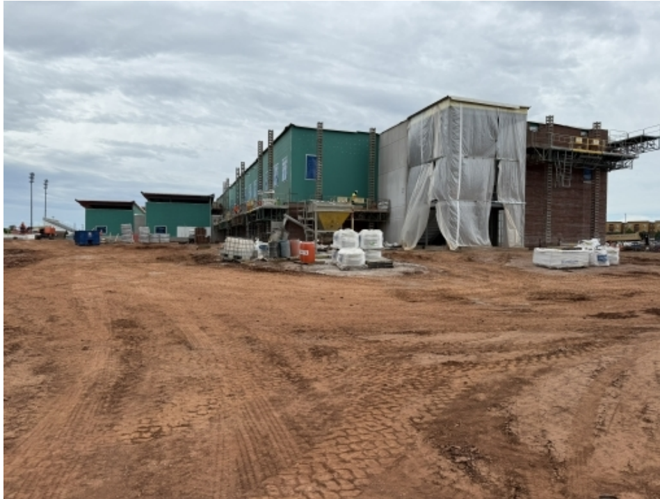
AREA 1 – NE EXTERIOR BRICK SCAFFOLDING
