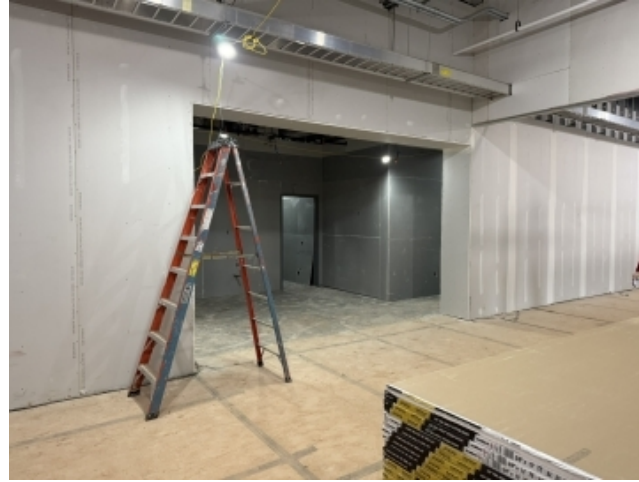
AREA 1 – RESTROOM ALCOVE
