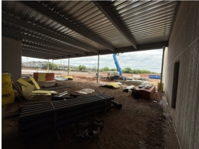
AREA 2 – SPED COVERED COURTYARD / PATIO AREA
