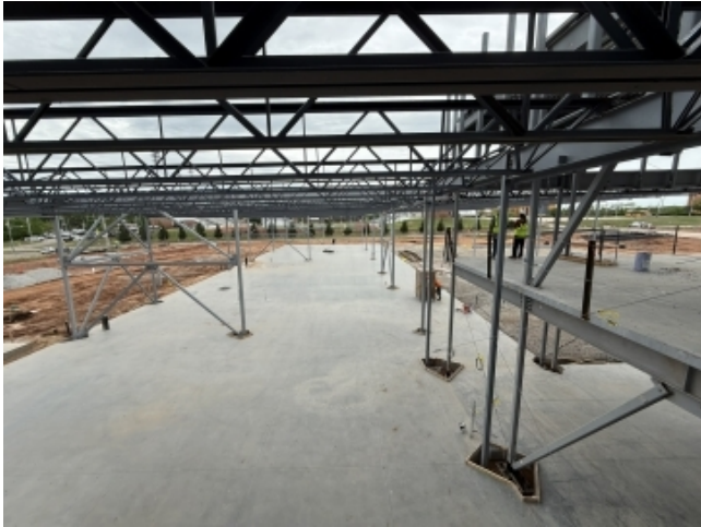
AREA 5 – STEEL ERECTION AND SLAB
