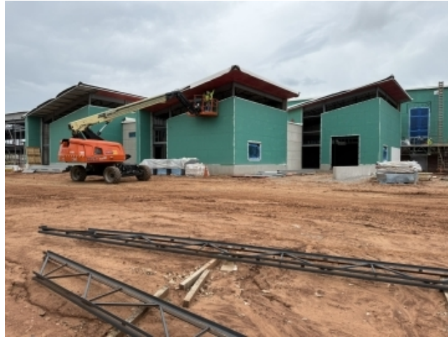
AREA 3 – VISUAL ARTS WING EXTERIOR
