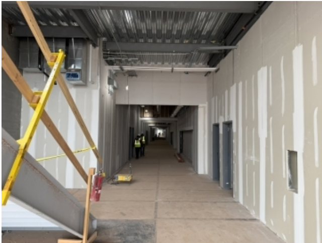
AREA 1 – NORTH STAIR / HALLWAY
