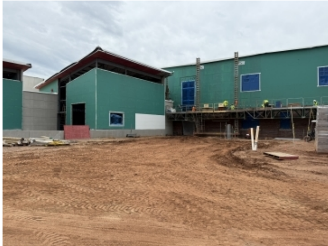
AREA 3 – VISUAL ARTS WING EXTERIOR
