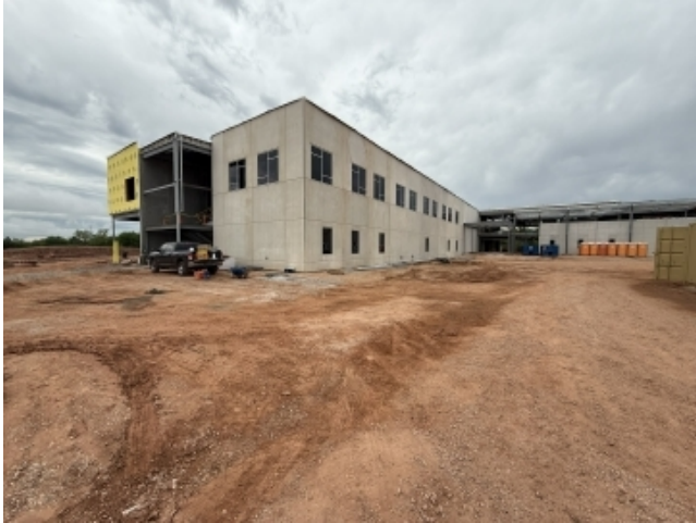
AREA 2 – EXERIOR PRECAST WINDOW INSTALLATION
