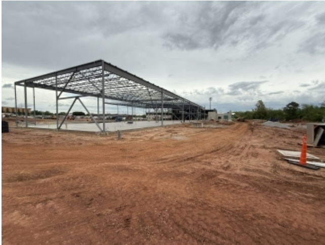
AREA 6 – STEEL ERECTION EAST SIDE
