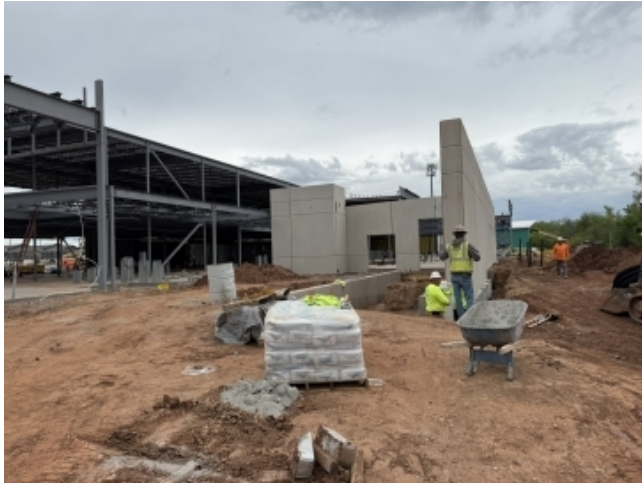
AREA 5 – LOADING DOCK PRECAST
